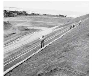
When under the pressure of severe conditions, even the best erosion control products can't function to their full potential without proper installation and anchoring. North American Green supplies a wide variety of fastener options for nearly every application and soil type.
