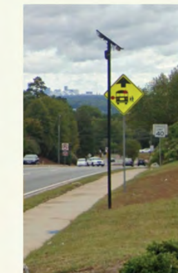
Solar & Flock Pole
