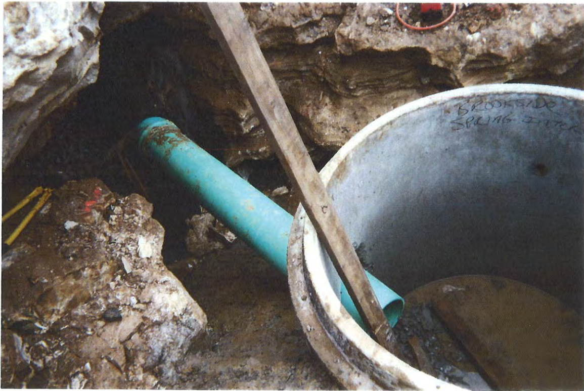
Photo 7. Installation of Perforated Drain.
