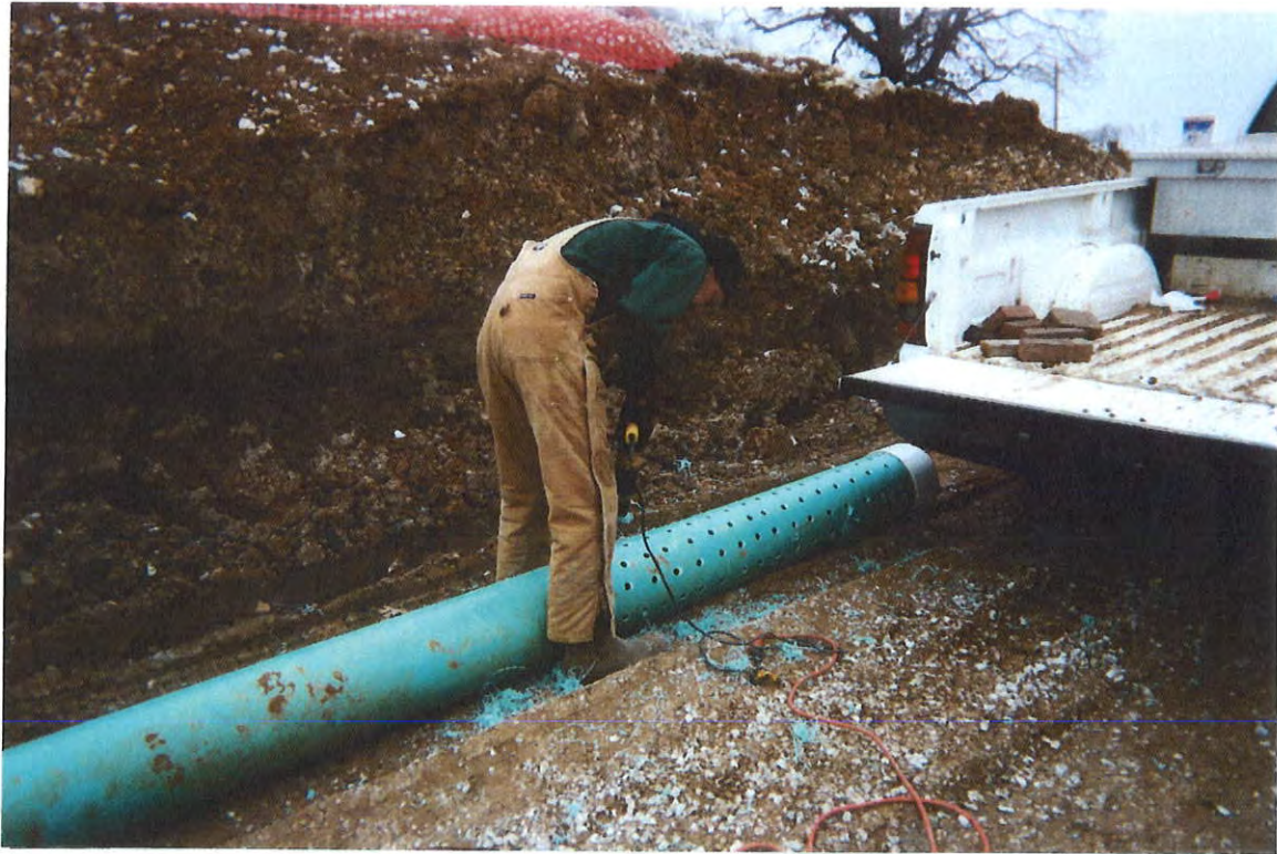
Photo 6. Construction of Perforated Drain.
