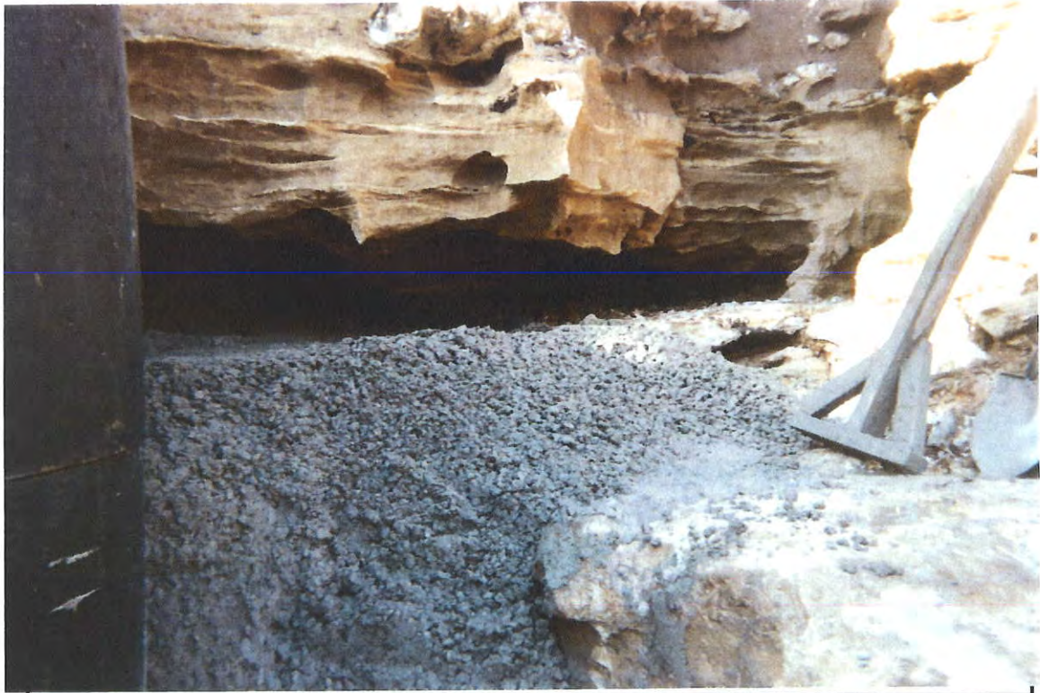
Photo 12. Concrete cap to bedrock shelf.
