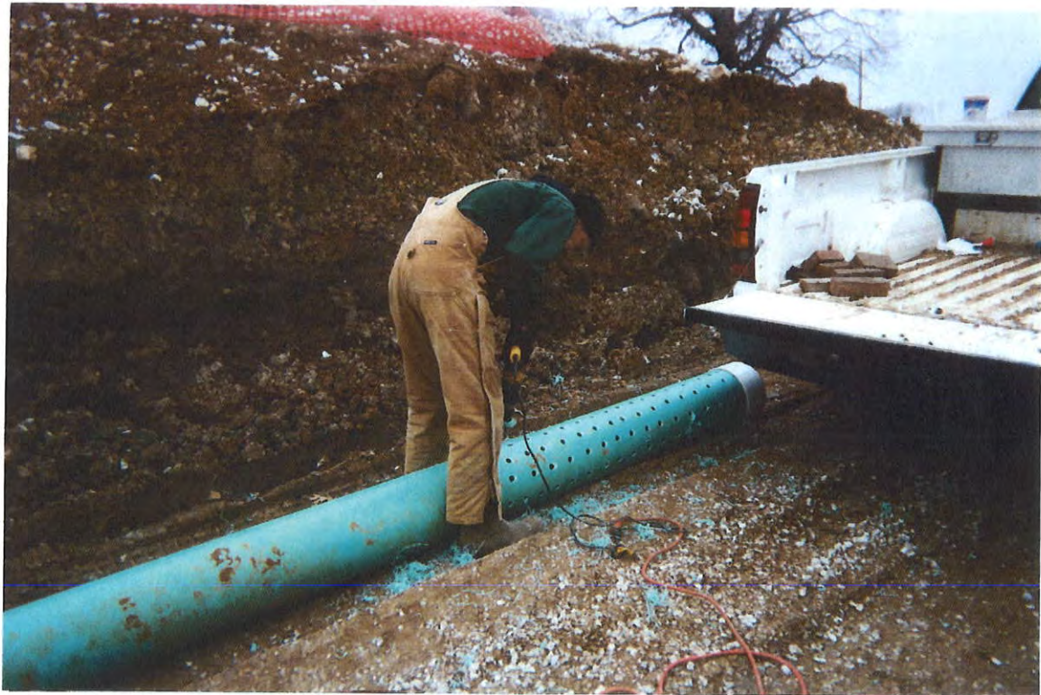
Photo 6. Construction of Perforated Drain.
