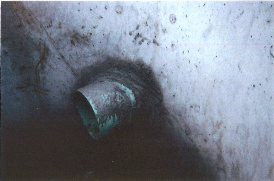
Photo 9. Spring drain into manhole.
