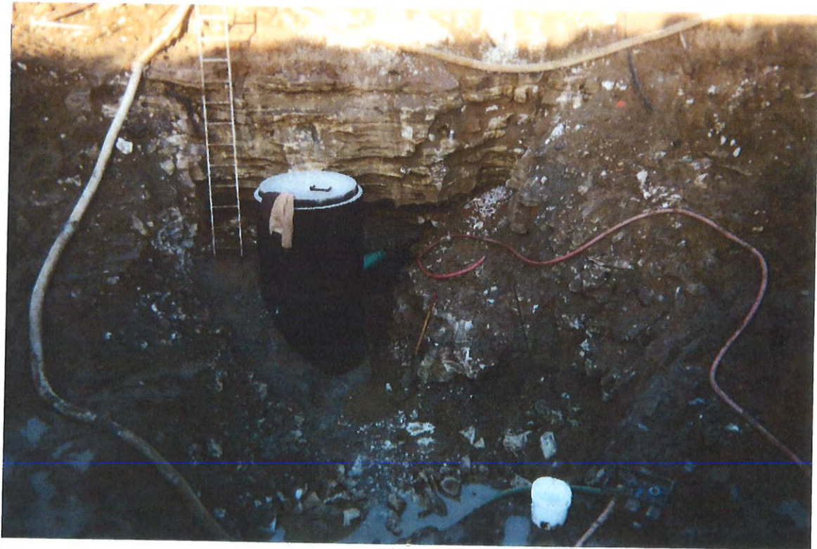
Photo 10. Overall view of Spring Interceptor.
