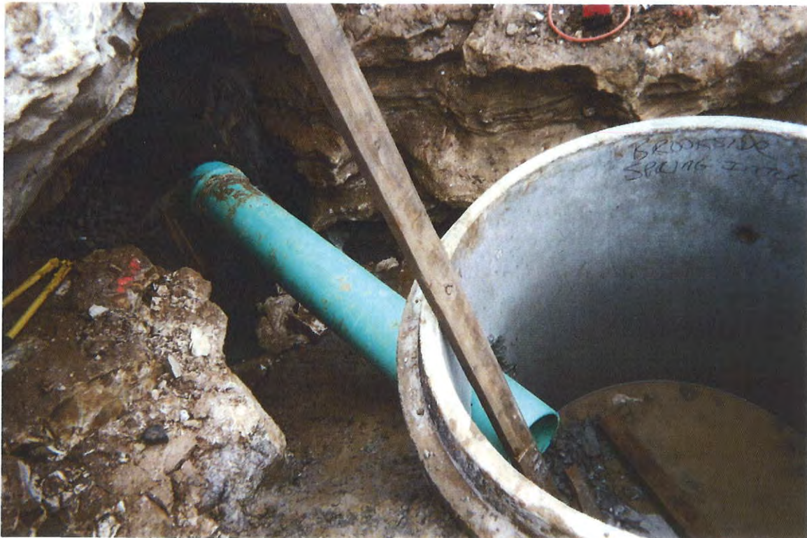
Photo 7. Installation of Perforated Drain.
