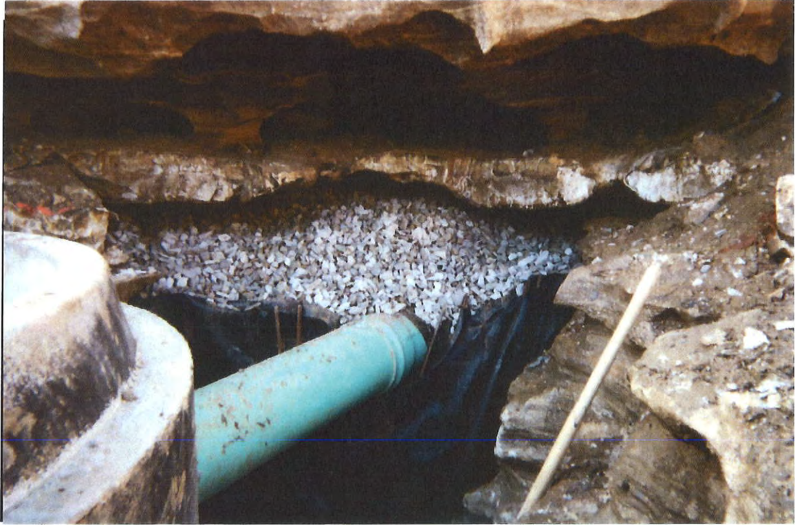
Photo 8. Clear rock backfill ground perforated drain.
