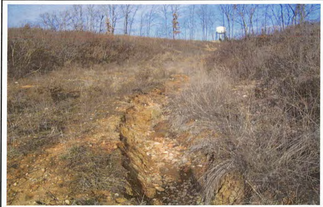
Photo 3. Eastern drainageway with erosional gully, facing north.
